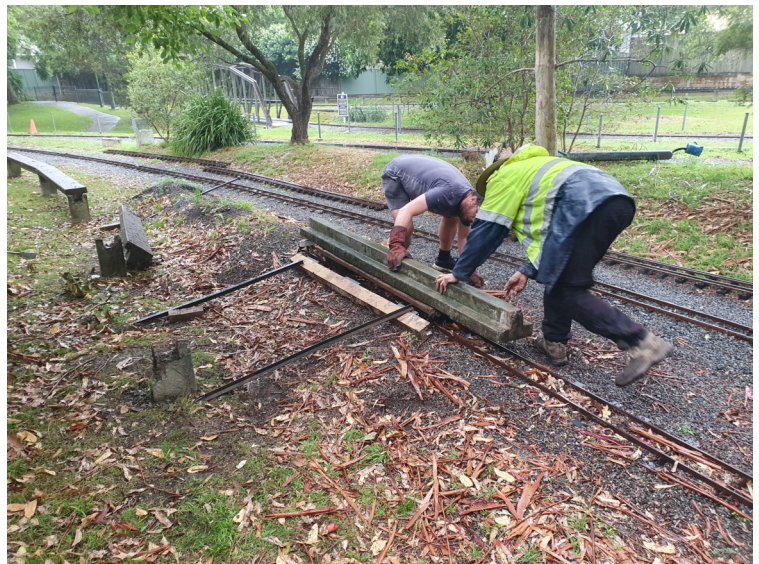
Above: Beam removal was a very quick affair. Here Chris and Andrew slide a beam onto a service car for delivery by rail to the disposal area. Below: The team march the first of the new channel sections into position. Note the raincoats.
